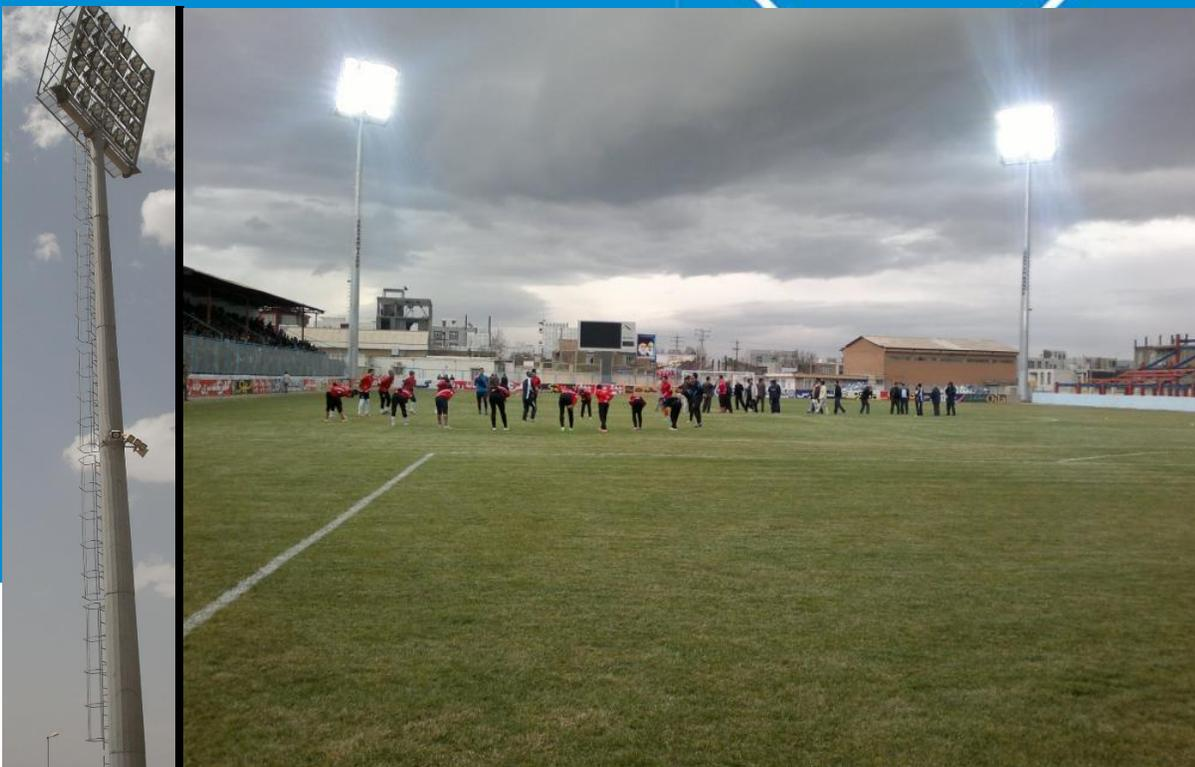
These structures are utilized in fixed and movable basket types. In the movable type, in order to replace or repair the light source, the basket is moved by an electric control fixed down the tower and the mechanical force of the motor. The easy and cheap movable type service and maintenance because of its movable head and no need for cranes for replacing lamps are some advantages of these structures.
