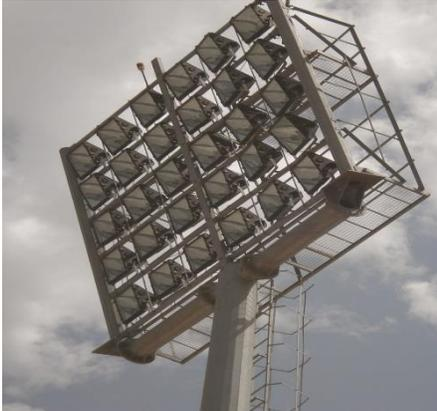
Stadium towers and structures are designed and produced to illuminate sports fields at different heights. The design of these poles is based on the type of the gymnasium application, required luxes of light regional atmospheric conditions, number of spectators, area and so on. A uniformly lighter and safer environment for spectators and players is a major objective of the design.
