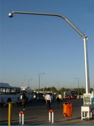
Traffic cameras which record the events and send the records to the traffic control center are among the most important and quickest ways of traffic monitoring.
